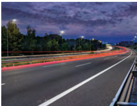
Madrid: street lighting
